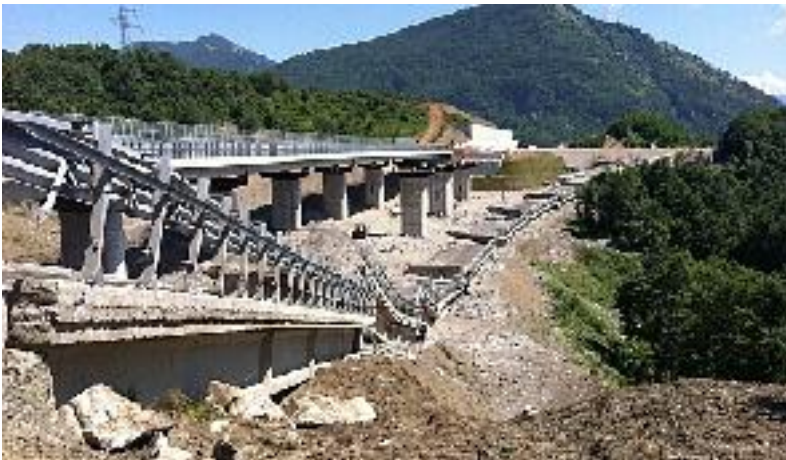
Figure 2: viaduct of figure 1, after having been cut down by pylons demolition.
