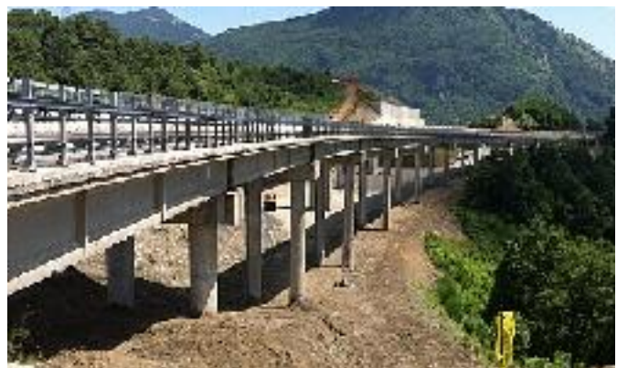
Figure 1: a viaduct to be demolished, with its 32 m (105 ft) long decks standing on 2 cylindrical pylons.
