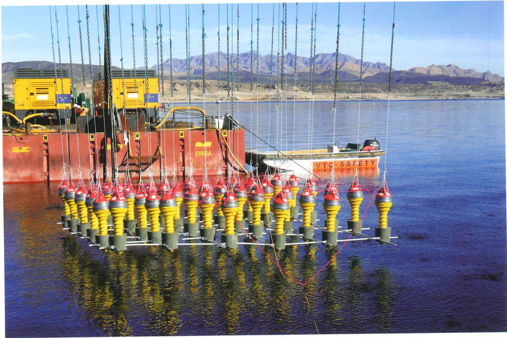
FIGURE 4.14 Lowering a field of shaped charges to the excavation site.
