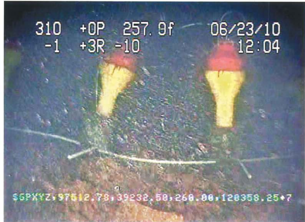
FIGURE 4.16 ROV screenshot of shaped charges resting on the surface of the excavation site.
