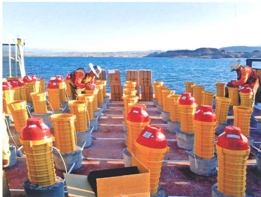
FIGURE 4.12 Shaped charges being prepared on the blasting barge.
