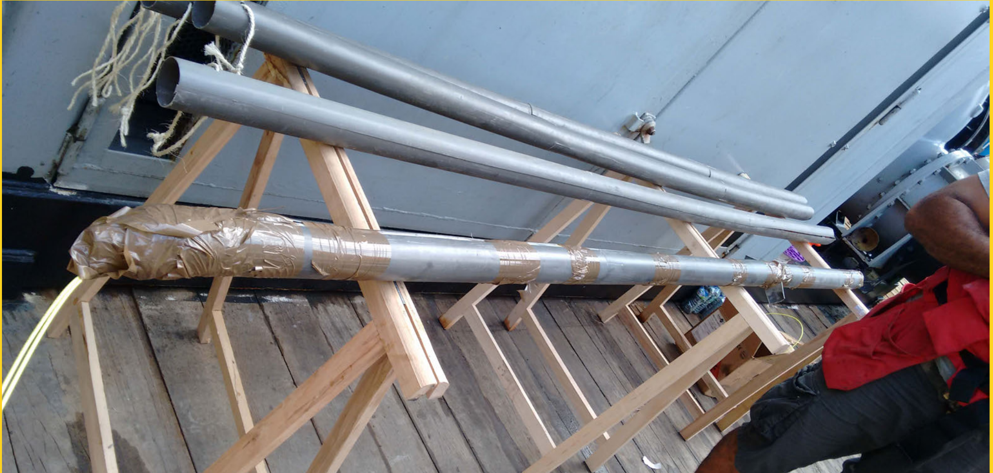
Explosives charges assembly into PVC pipes, including ballast and stemming
