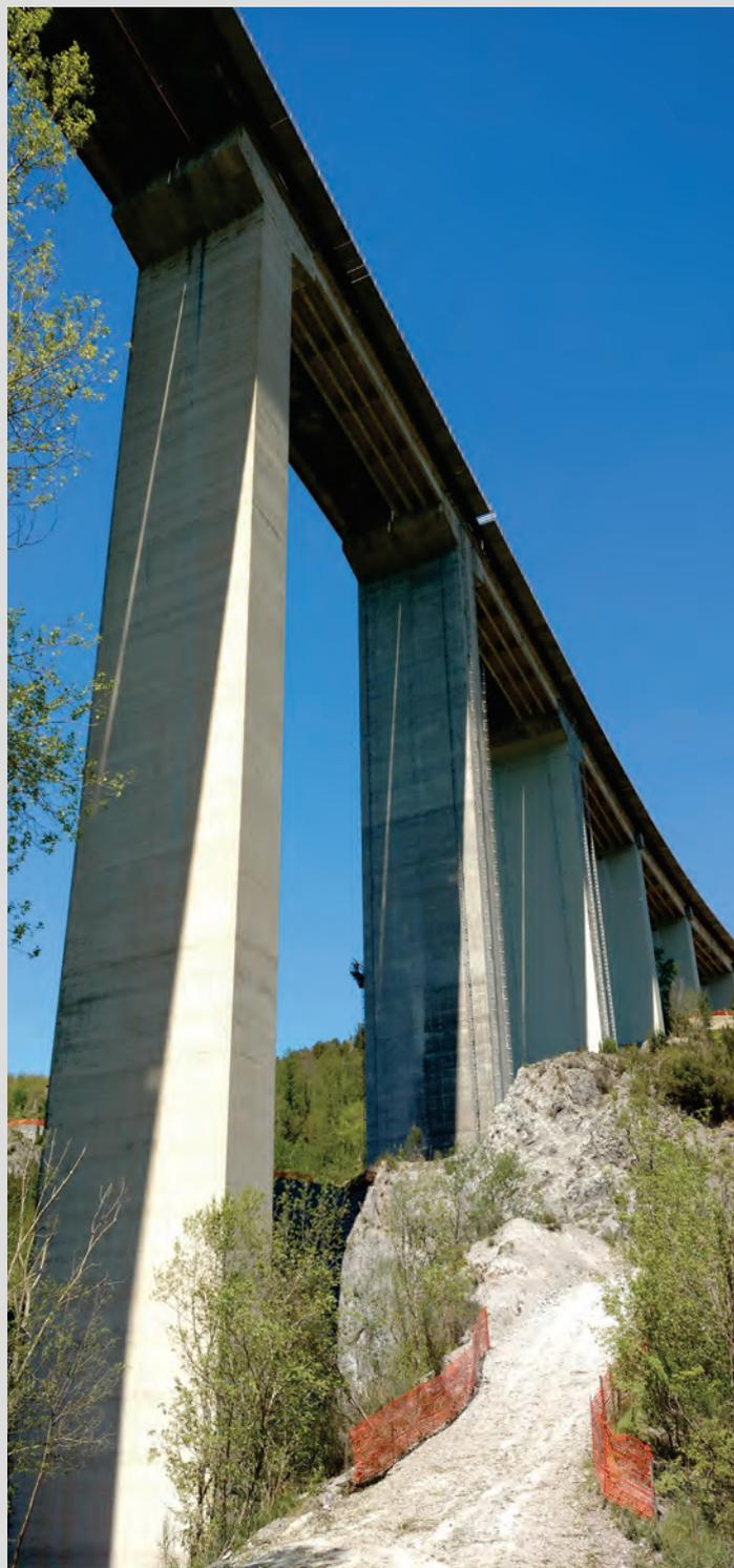
Customer: **ITALSARC S.C.p.A.**Site Job: **Laino Borgo, (Cosenza), Italy – A3 SA-RC Highway**Date: **2014 - 2016**The **JANNELLO** bridges: 22 spans 45 meters long, I beams, 20 pylons to be safeguarded.
