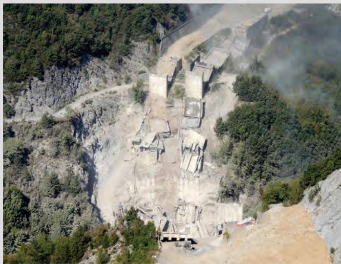
Customer: **ITALSARC S.C.p.A.**Site Job: **Laino Borgo, (Cosenza), Italy – A3 SA-RC Highway**Date: **2016**The **BATTENDIERO I** bridges: 16 spans 35 meters long, I beams, 14 pylons to be tilted down.
