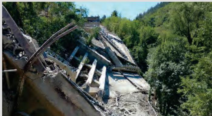
Customer: **ITALSARC S.C.p.A.**Site Job: **Mormanno, (Cosenza), Italy – A3 SA-RC Highway, year 2016.**The **SAN MICHELE** bridge: 4 spans 32 meters long, I beams, 3 pylons to be tilted down.
