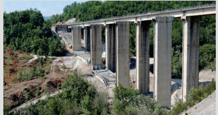
Customer: **CARENA spa**Site Job: **Lauria, (Potenza), Italy – A3 SA-RC Highway. Date: 2012- 2014**The **MACERA 2** bridges: 18 spans 32 meters long, I beams, 16 pylons to be safeguarded.
