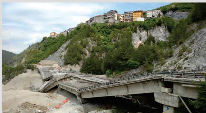
Customer: **ITALSARC S.C.p.A.**Site Job: **Mormanno, (Cosenza), Italy – A3 SA-RC Highway, year 2016.**The **LA PINETTA** bridges: 14 spans 32 meters long, I beams, 12 pylons to be tilted down.
