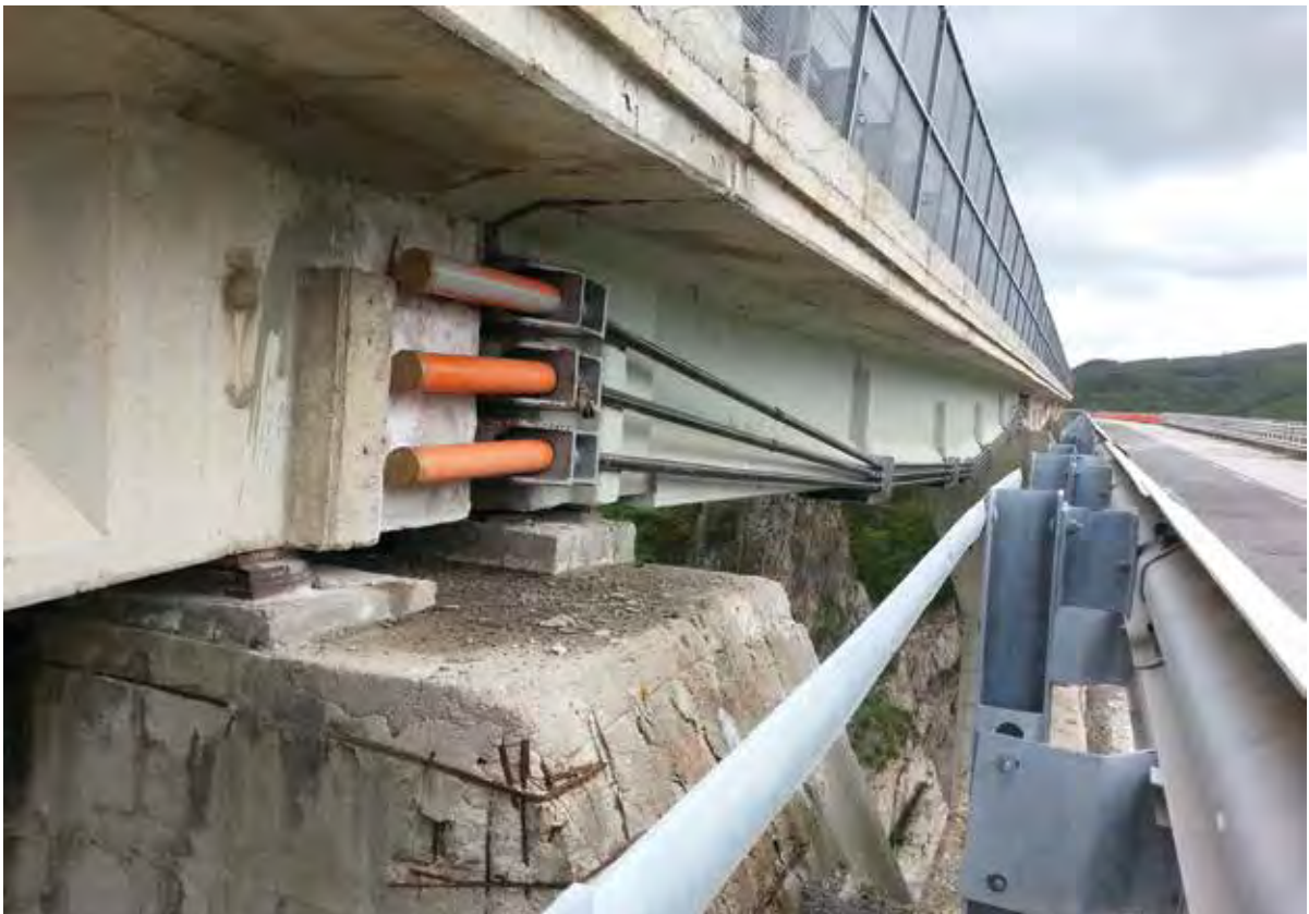
Figure 4. Northern (left, to be left in place in service) and Southern carriageways of the Pietrastretta bridge.
