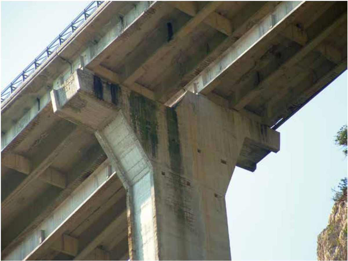
Figure 3. Detail of the cantilevers supporting the two carriageways and of the post-tensioned transverse beams tying together the three main beams.
