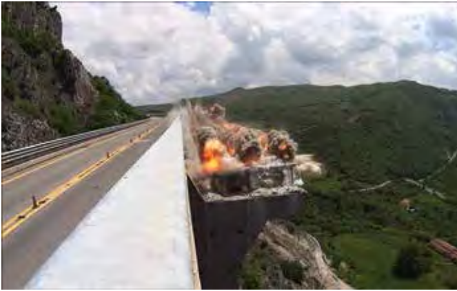
Figure 24. Sequence of blasts.
