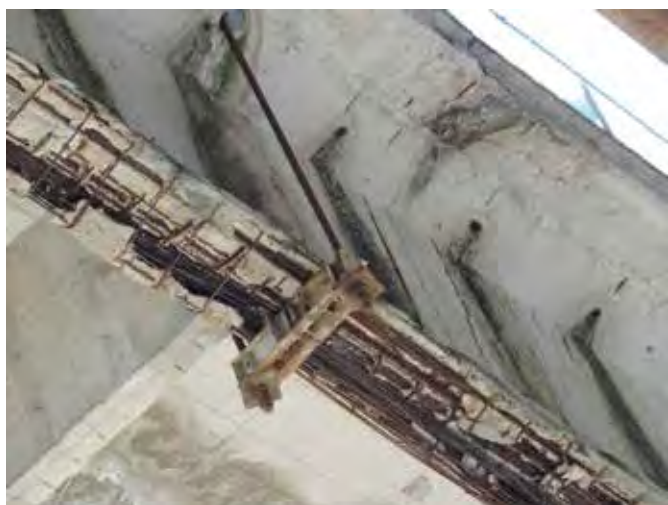
Figure 8. Detail of degradation.
