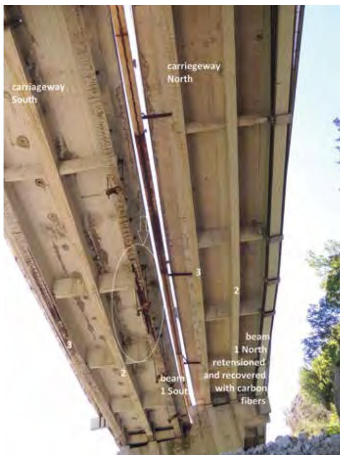
Figure 7. Strong degradation of the beams at 12th span southern carriageway, lower flange, with lost of concrete layers, extended corrosion and broken re-bars and tensioning wires.
