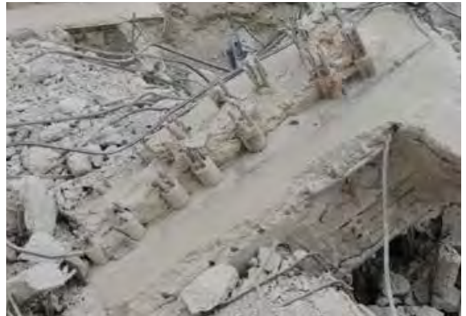
Figure 23. Detail of the tensioning heads being exposed after the blast.
