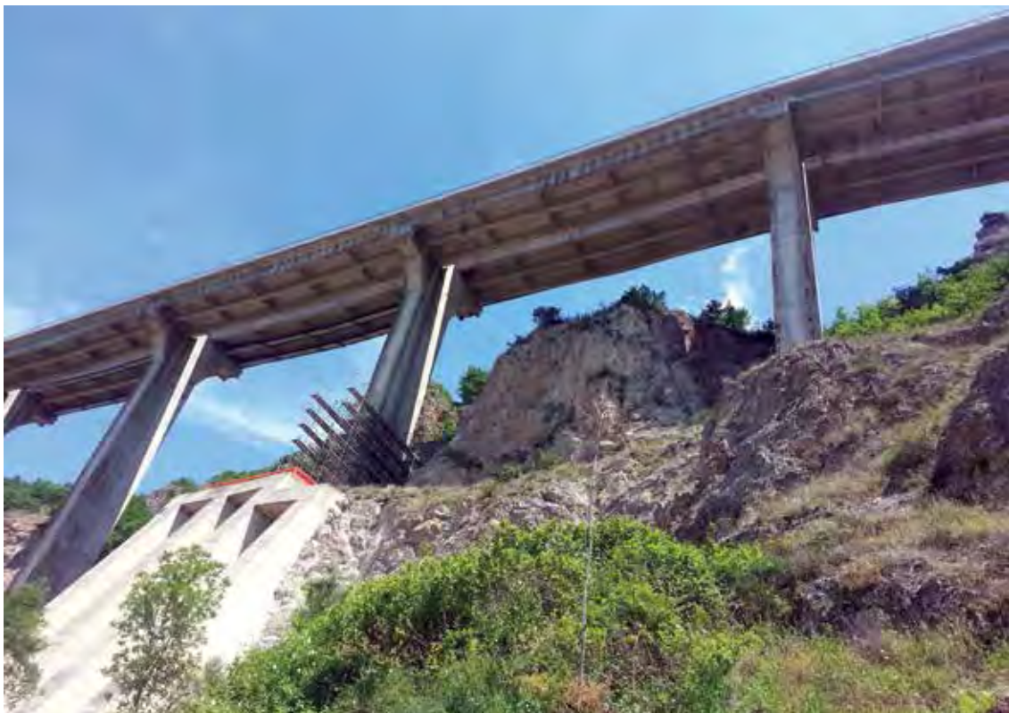
Figure 2. Detail of the bridge.
