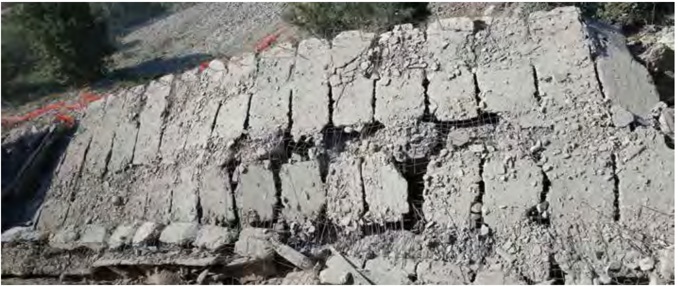
Figure 21. Span blasted in one single-step at the ground.
