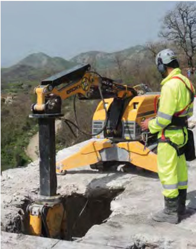
Figure 16. Cut of transverse beams by means of a hydraulic crusher on a remote-controlled electric excavator.
