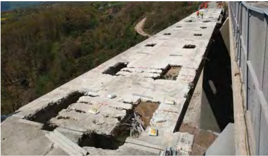
Figure 18. Span prepared and loaded for triple-step blasting.
