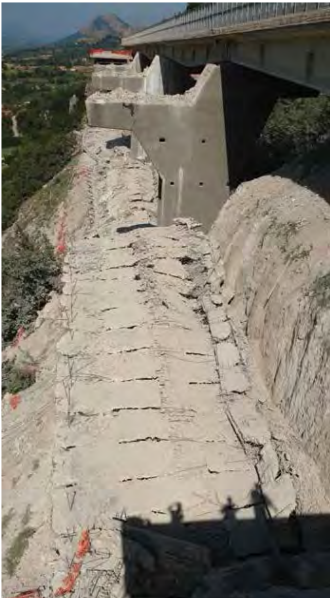
Figure 22. Several spans blasted in one single-step at the ground.
