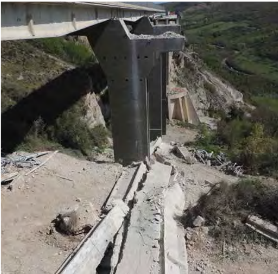
Figure 19. Span blasted in triple-step at the ground.
